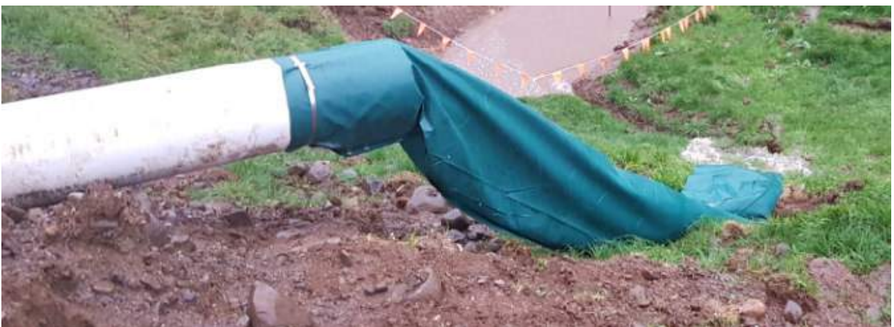
Figure A 7: Aqua Duct – drop structure photo
